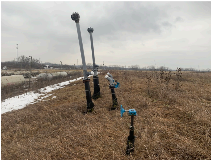
Photo 14 : Gas vents along east side of property
